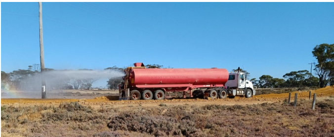
Above and below: Slarke St road works
