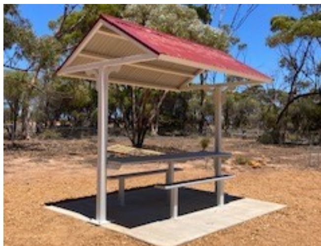
Installation of a shelter at the Newdegate Cemetery
