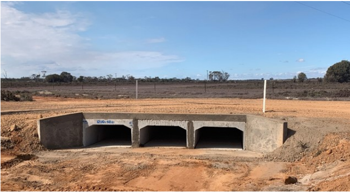
Above: Slarke Street Drainage Upgrade
