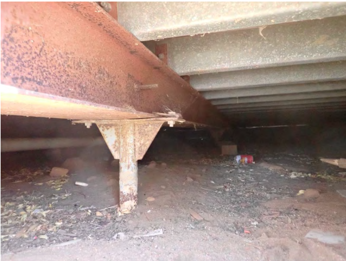
Figure 9: Steel joists, bearers and stumps.
