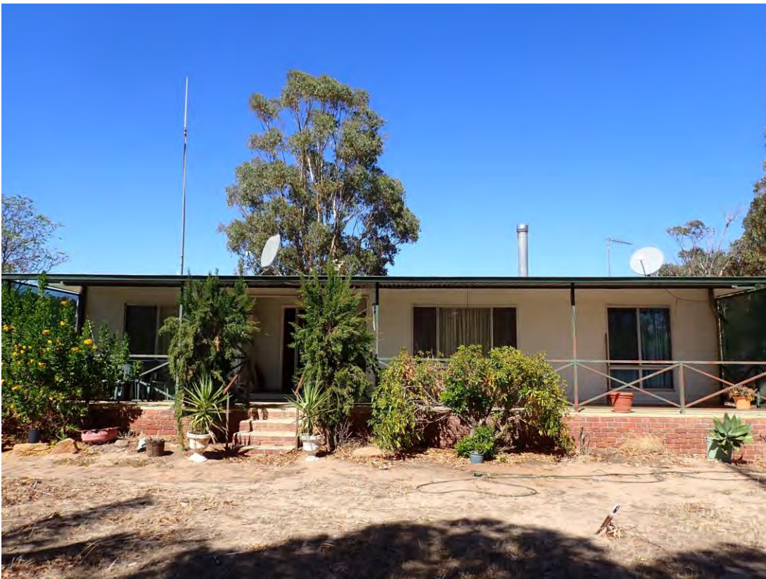
Figure 3: Photo of North Elevation
