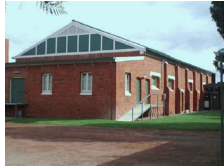
Rear side loading door and ramp
